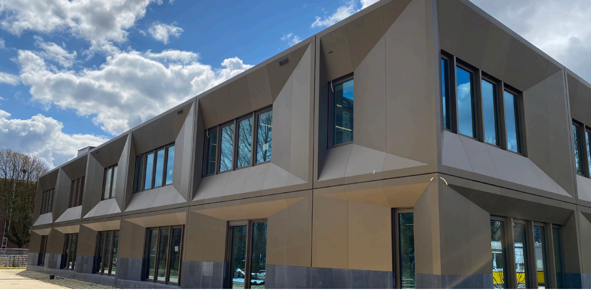
Image: © Compal Composites Photo of the Alucobond facade of the „Praktijk College in Rotterdam“
